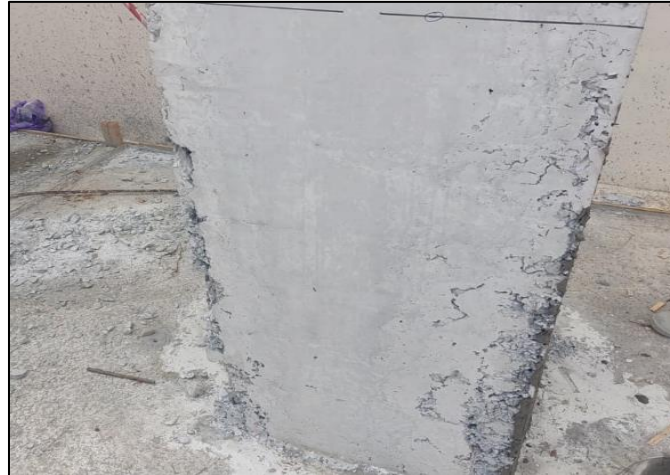
Gambar 1. Beton Honeycomb
